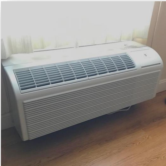
Packaged Terminal Heat Pump
